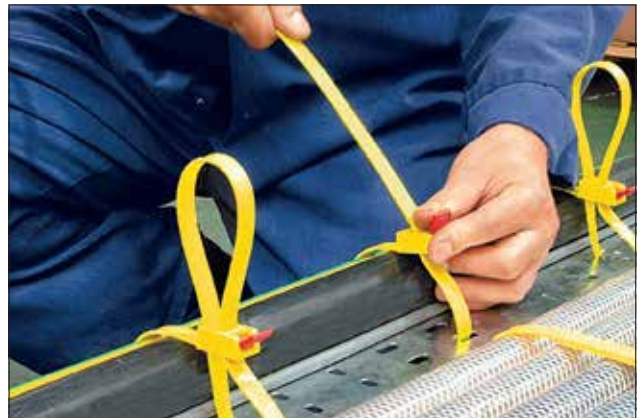
Excess tails can be neatly tucked away.
