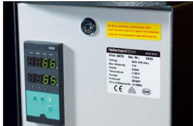
Professional type plate on a heating unit.
