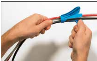
Insert one or more cables into the insertion slot of the HAT applicator tool.
