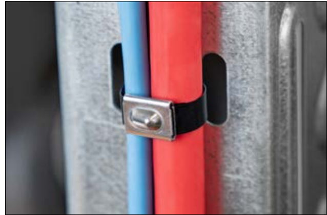
Stainless steel cable ties, coated, MBT_SFC, MBT_HFC.
