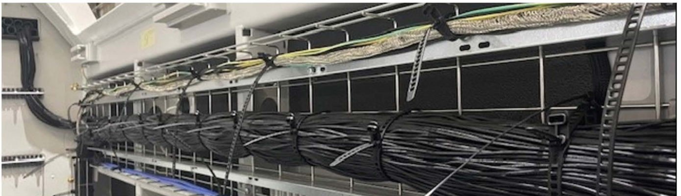
Secure bundling of heavy cables during assembly
