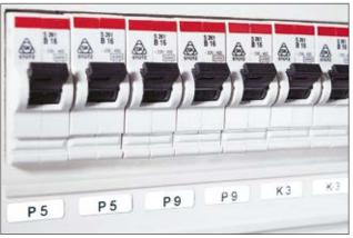
Clear and permanent identification of switch gears.
