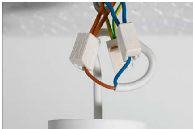
Quick installation and release of lighting devices with HelaCon Lux.
