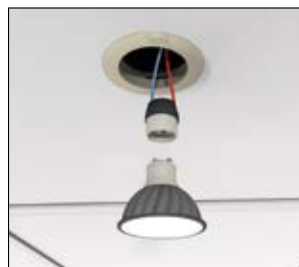
3. Connect the bulb to the socket and lock into the correct position.
