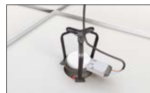
4. Connect the downlight to the power supply and fix the cable into the routing eyelet.
