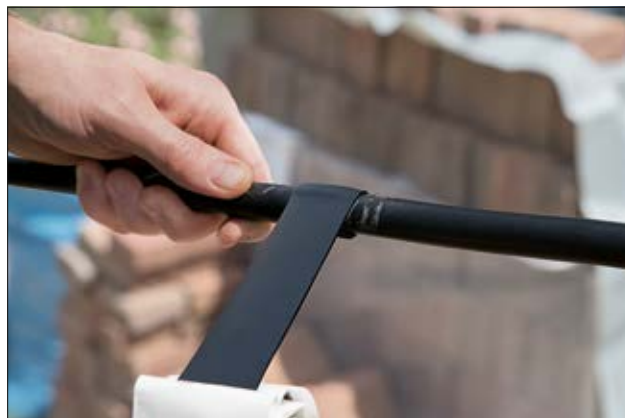
HelaTape Power self-amalgamating mastic is highly flexible.
