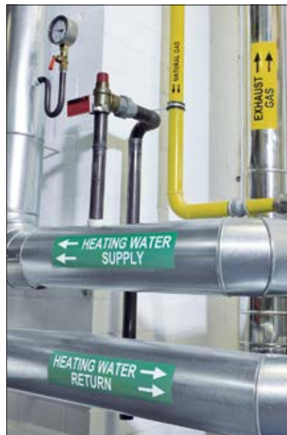
Large and highly visible pipe marking.
